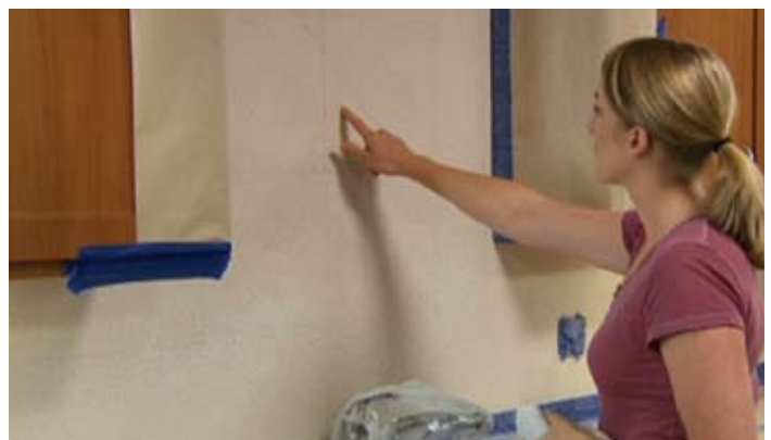
Be sure to test the wall with your finger before setting tiles.
