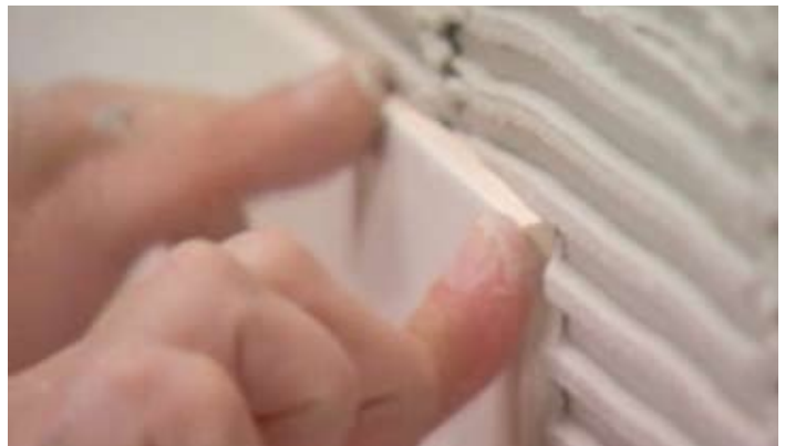
Press the tile into place and slide it across adhesive ridges.
