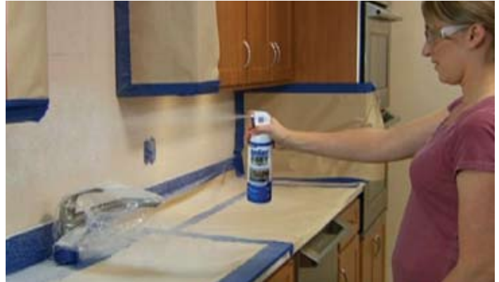
While spraying, hold the can at least 18"- 24" from the wall surface.
