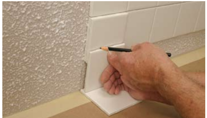
When cutting a tile be sure to measure carefully.
