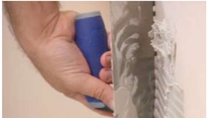
When applying adhesive, make certain the teeth of the trowel touch the wall.
