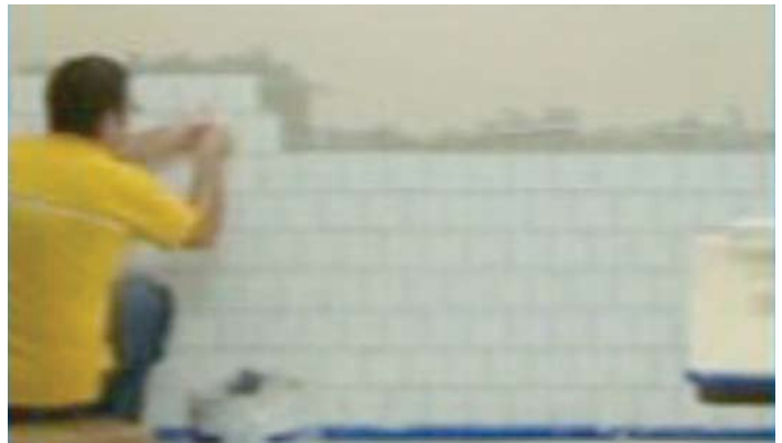
Thinset or mastic may be good choices for damaged, uneven walls.
