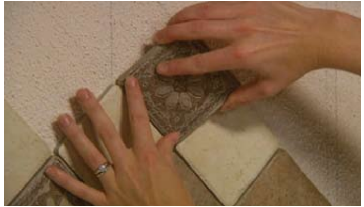
Tip the tile into place – do not slide or wiggle tiles.
