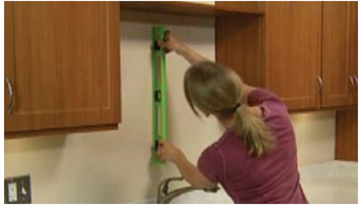
Be sure to carefully check your wall surface.
