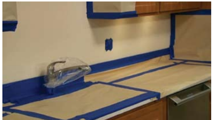
Be sure to mask off the area to protect surfaces.
