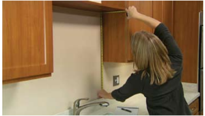
Measure your wall carefully to determine square footage.
