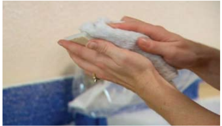
Be sure to clean and dry tile backs.
