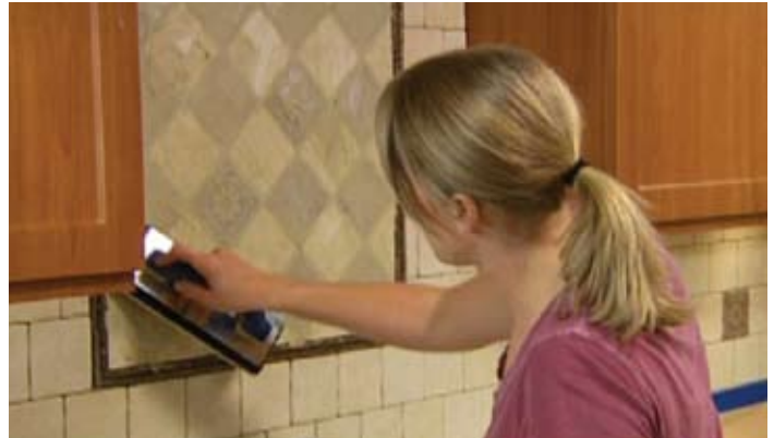
Use a rubber grout float to apply your grout.
