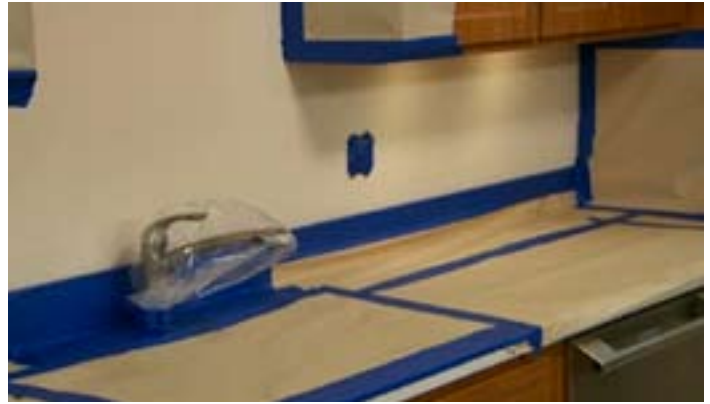
Carefully prepare the work area before setting tile.
