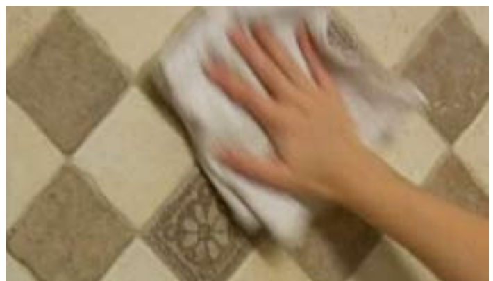
Remove haze with a damp rag, then a clean, dry rag.
