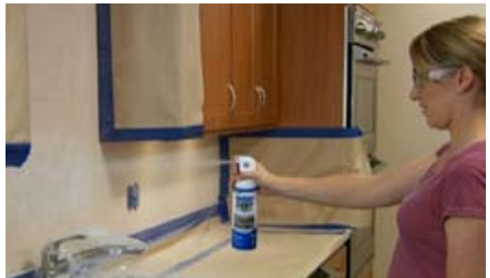
Be sure to hold the can 18" to 24" from wall when spraying.
