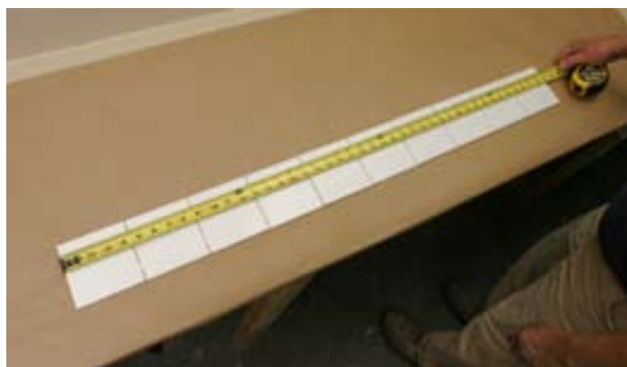
Lay out your tiles and measure carefully to determine each tile's length with grout lines.
