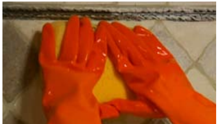
Once set, clean the tile with a damp sponge – rinsing it often.
