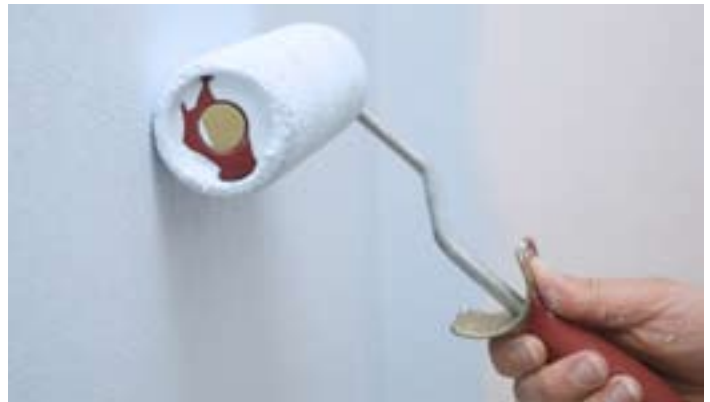
Sheet rock should be primed and/or painted with latex paint.
