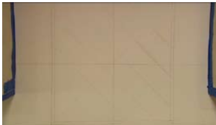
A proper grid pattern will help prevent tiling mistakes.
