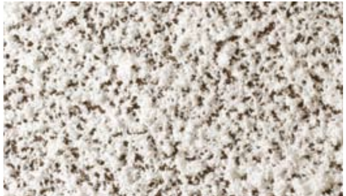
This is what a properly sprayed wall looks like immediately after spraying.
