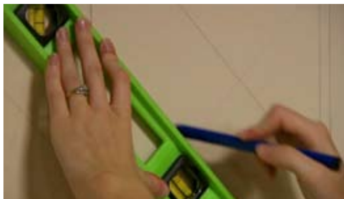
Use a level to carefully layout your grid.
