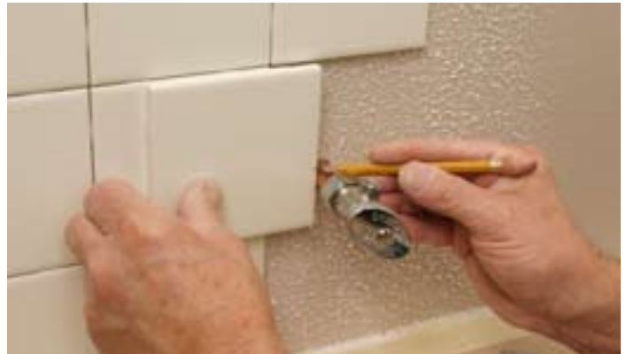
Mark holes by holding the tile over previously set tiles.
