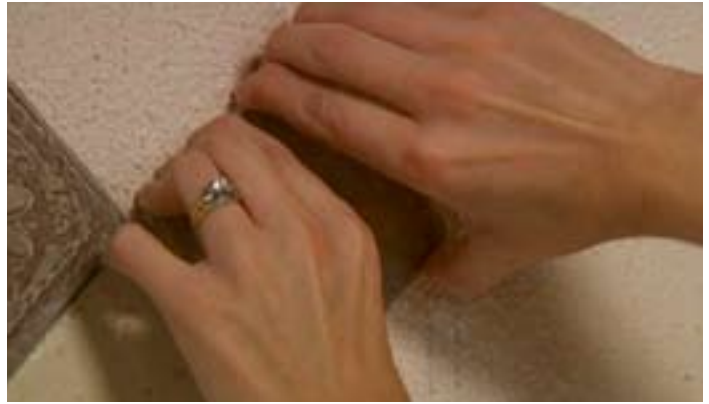
To remove a tile, pull it back and down from the wall.
