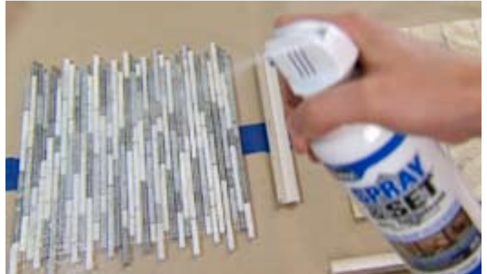
Be sure to apply a light coating (back-buttering) to mesh-backed tiles.
