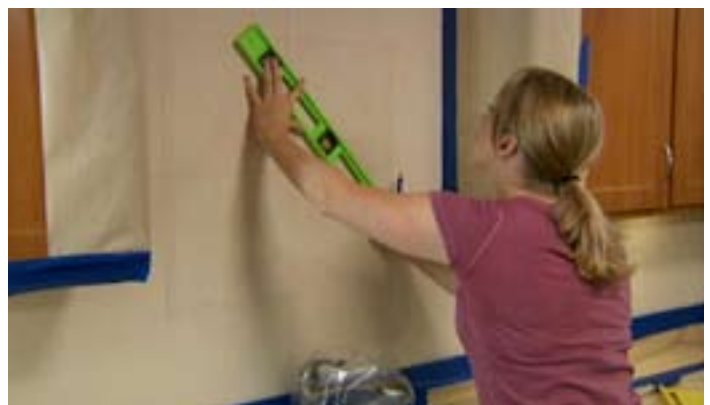
Lay out a grid pattern on your wall before setting tiles.
