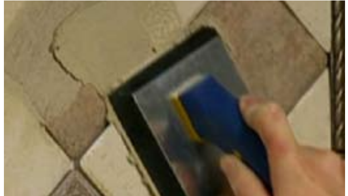
Press the grout into all joints using several sweeps.
