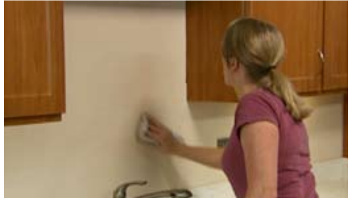
Walls must be clean and dry before setting tiles.
